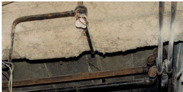
**Figure 48b** Poorly tamped sprayed chrysotile fireproofing on a structural steel beam holding up a concrete floor, showing some overspray onto the concrete and damage by electrical work
