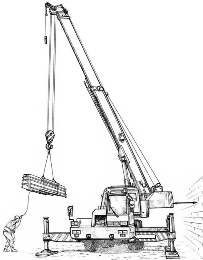
**Figure 40** A mobile crane is supported on outriggers which are prevented from sinking into the ground by timber packing. The crane is positioned to ensure adequate clearance between the wall and the counterweight. The slings are protected by packing around the load. The load is fitted with a tag line to allow it to be easily controlled
