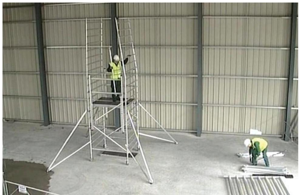
**Figure 11** Advanced guard rails
