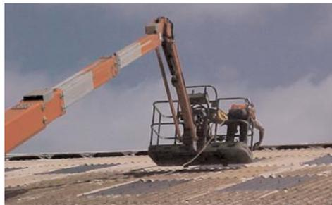
**Figure 26** A mobile elevating work platform being used to replace a roof sheet
