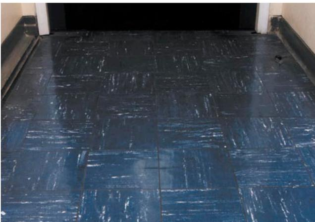
**Figure 48e** Asbestos-containing vinyl floor tiles
