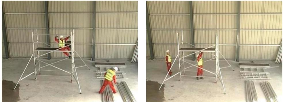
**Figure 12a and b** Through the trap
