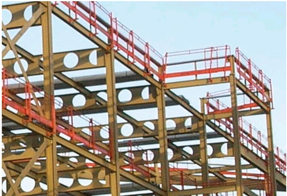
**Figure 28** Edge protection installed with the steelwork
