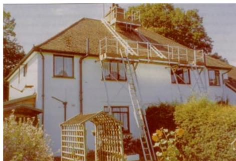
**Figure 25** Proprietary access system for roof-work
