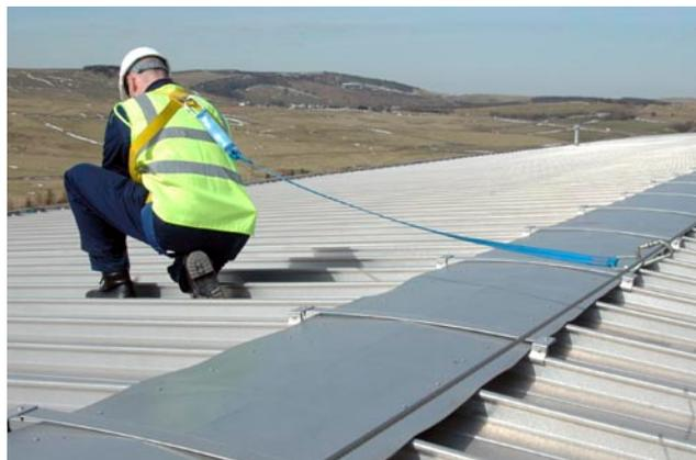
**Figure 16** A work-restraint harness
