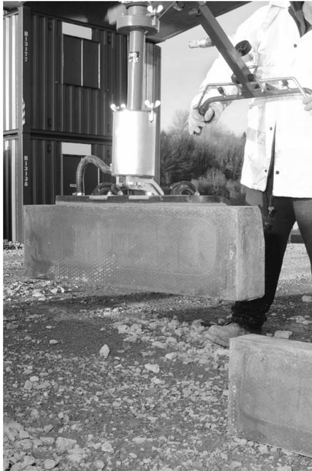
**Figure 38** Handling kerbs using a vacuum lifter
